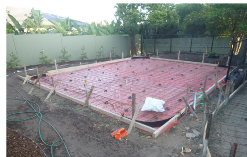
Parratt residence; retaining wall and court construction, including painted fences
