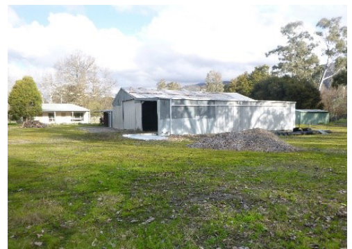
Kiewa River community park site; existing conditions
